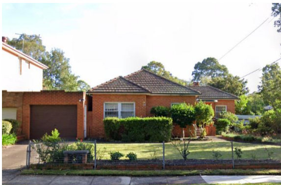
Figure 36: 59 Hallam Street, Lane Cove West (Constructed 1943-1951) (Source: Google Maps, Mar 2020)
